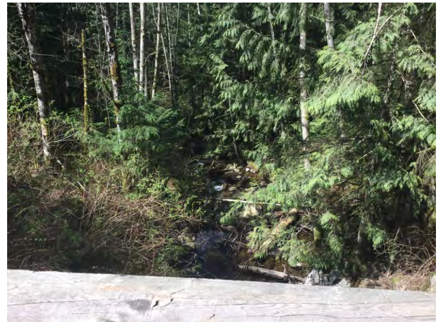
Looking downstream from deck
