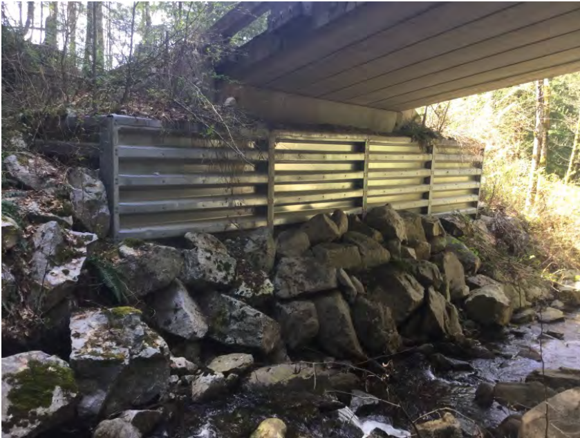
Left Bank Abutment when facing downstream
