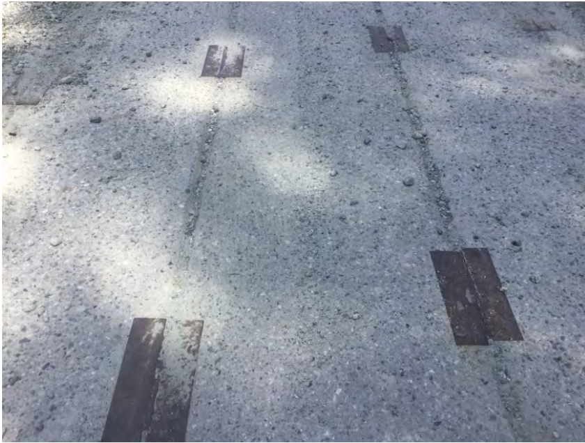
Welded shear connectors - typical
