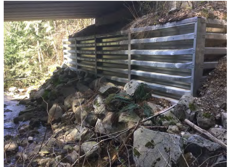
Right Bank Abutment when facing downstream
